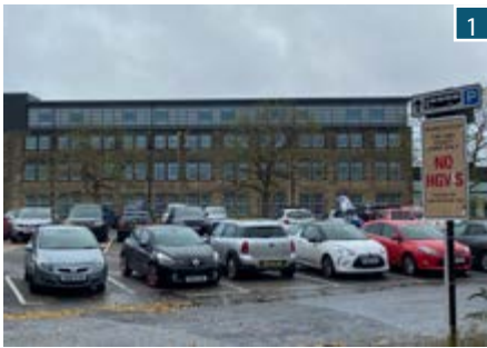
St. Leonard's Gate car park.
