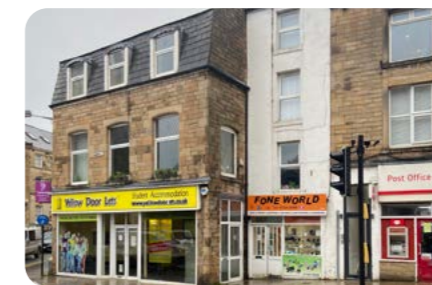
Potential for new pedestrian access through no.2 Stonewell.
