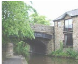
Nelson Street Bridge
