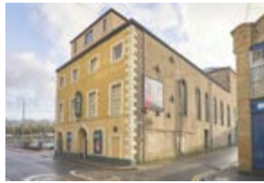
Georgian society: Grand Theatre (1781). Rendered sandstone rubble, slate roof. Main facade has chamfered quoins and is of 3 storeys and 4 bays.
