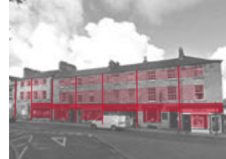
Dalton Square west side: Late 19th century ground floor timber shop fronts form strong horizontal plinth on top of regular vertical glazed bays. Three storey, two bay former residential buildings (Georgian).
