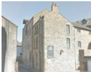
18th C warehouses, Dye House Lane
