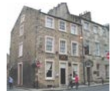
Inns were built to serve travellers between England and Scotland. The Sun Inn, Church Street (1785). Georgian period building of rubble faced sandstone.
